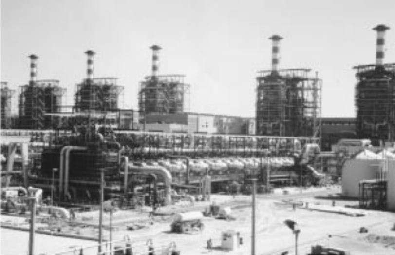
**FIGURE 20.6.2** One of the six units of the 346,000 m<sup>3</sup>/day MSF desalination plant Al Taweelah B in Abu Dhabi, United Arab Emirates. (Courtesy of Italmimpianti S. p. A.) It is a dual-purpose plant, composed of six identical power and desalination units. Five of the six boilers are seen in the background. The desalination units were in 1996 the largest in the world. They have 17 recovery and 3 reject stages and a performance ratio (PR) of 8.1. The plant also produces 732 MWe of power.
