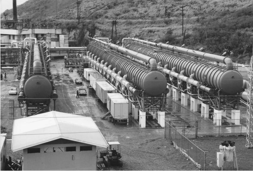
**FIGURE 20.6.3** Two HTME desalination units, each producing 5000 m<sup>3</sup>/day, in St. Croix, U.S. Virgin Islands. (Courtesy of I.D.E. Technologies Ltd.)
